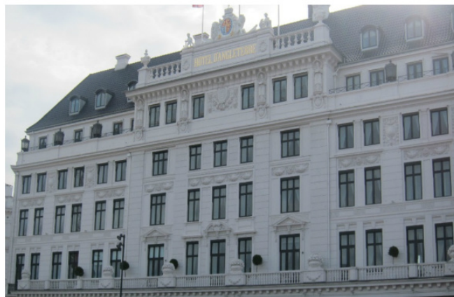
Hotel d' Angel Terre , photo taken by the author, Copenhagen, Denmark, 2015
